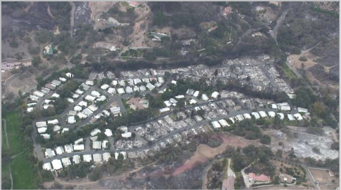
Destroyed mobile homes in the Valley Oaks Mobile Home Park following the Rice Fire in San Diego County (Source: ImageCat)
