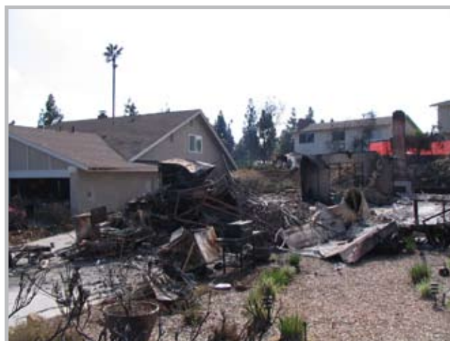
Burnt residential structure following the Witch Fire in San Diego County. As fire suppression crews fought to save the surrounding homes, this home burned to the ground. (Source: RMS)
