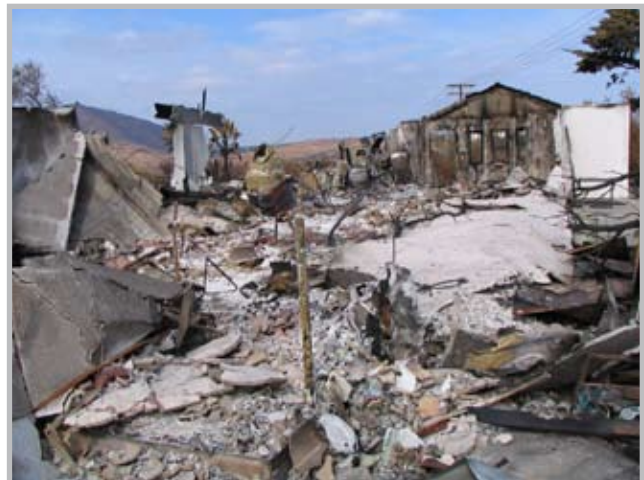
Destroyed residential structure along the wildland-urban interface as a result of the Witch Fire in San Diego County in 2007 (Source: RMS)
