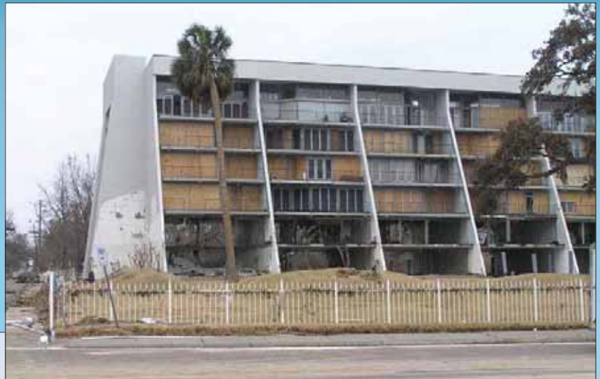
Figure 7. Storm surge damage to the lower stories of a reinforced concrete hotel in Biloxi, MS
