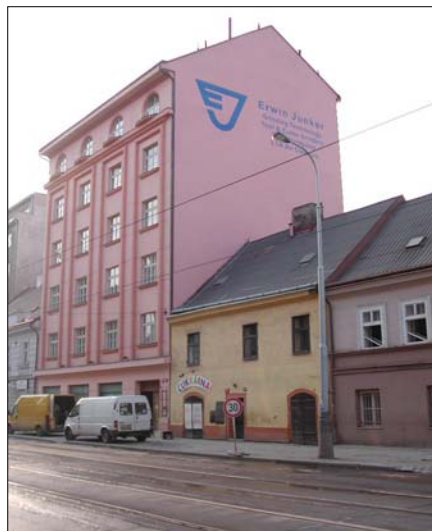
Figure 20. Water lines on these structures mark peak flood heights impacting the first two stories of properties in some portions of Karlin
