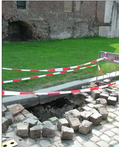
Figure 13. Repairs to below ground infrastructure were visible throughout the Old Town
