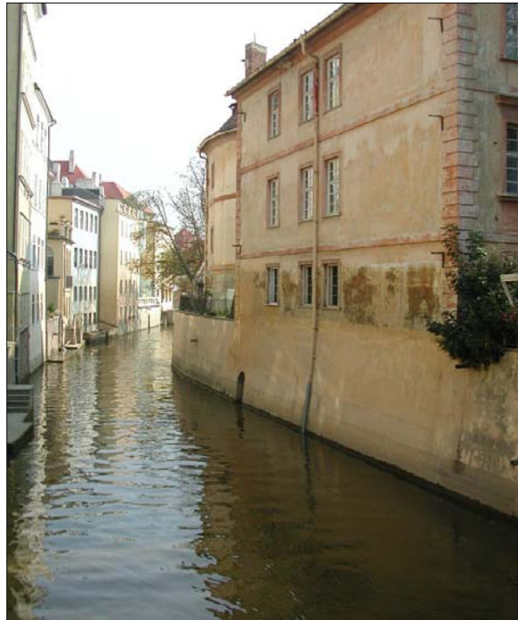
Figure 16. Water marks are clearly visible on the outside of this building on Certovka Creek, immediately west of Kampa Island
