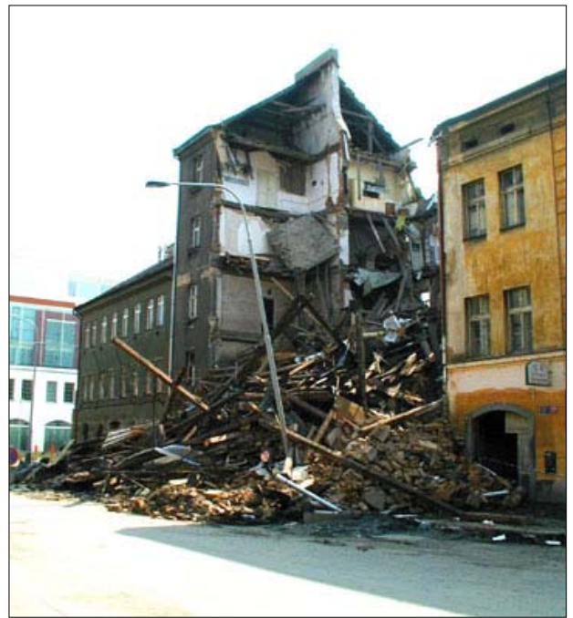
Figure 18. This multi-story building collapsed whilst the district was still flooded. The complete failure of one part of the building can clearly be seen (photos courtesy of Radio Prague)
