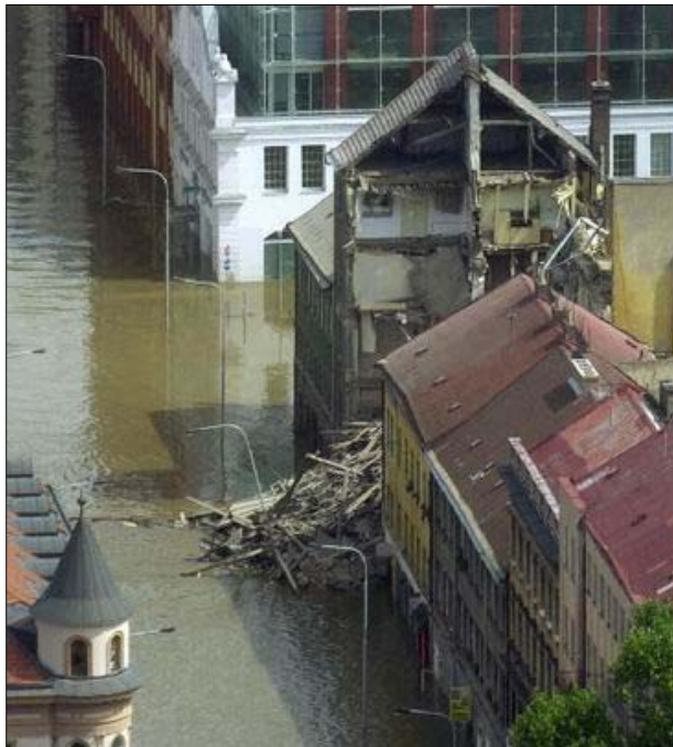
Figure 18. This multi-story building collapsed whilst the district was still flooded. The complete failure of one part of the building can clearly be seen (photos courtesy of Radio Prague)
