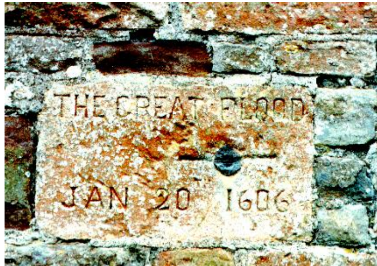
Figure 3: Stone on the wall of a local church in Peterstone Wentlooge (northeast of Cardiff) marking the height reached by the 1607 Bristol Channel Floods (about 1.9 meters 1 above ground level) and reading "The Great Flood Jan 20, 1606" (from Great Flood of 1607 website: http://website.lineone.net/~mike.kohnstamm/flood/ )
