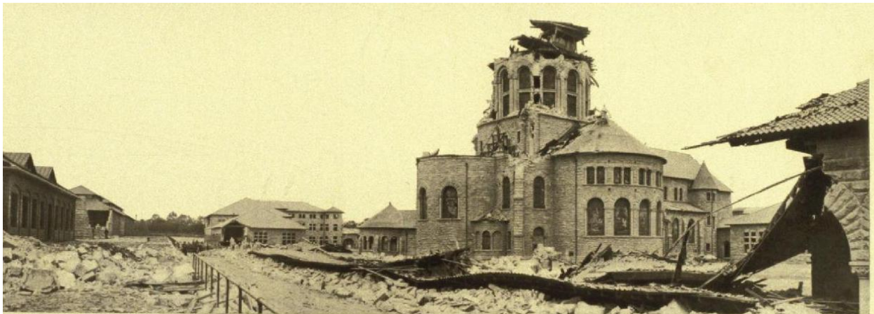
Figure 1: Damage at Stanford University following the 1906 San Francisco Earthquake (Source: Lawson, 1908)
