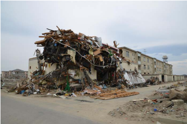
Figure 3: Damage (and debris) due to tsunami waves along the coastline near Sendai in Miyagi Prefecture (Source: RMS reconnaissance)
