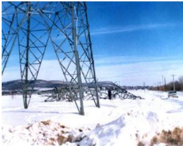
*Figure 5: Collapse of Hydro-Québec pylon during the 1998 Ice Storm (Source: [http://www.vancouverislandpowerline.com/quebec\\_ice\\_storm.html](http://www.vancouverislandpowerline.com/quebec_ice_storm.html) )*
