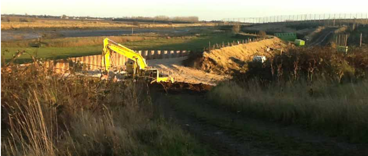
Figure 8: Repair work underway at the breached Boston Dike
