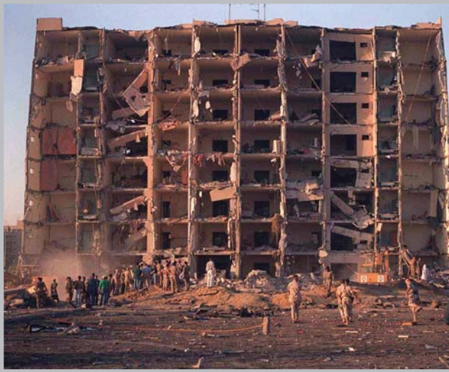
Terrorist attacks can be very ambitious and destructive as seen in the use of a large truck bomb against the Khobar Towers in 1996 causing the collapse of apartment buildings containing more than 3,000 occupants at a U.S. Air Base in Saudi Arabia (Source: U.S. Department of Defense)
