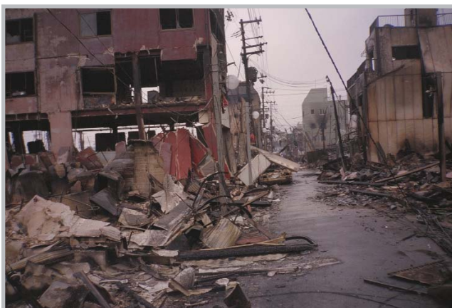
Fire following earthquake can significantly increase damage and casualties, as seen in this neighborhood ravaged by fire by the 1995 Kobe Earthquake
