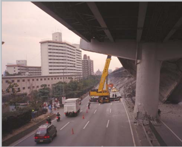
Other earthquake-related catastrophes such as a collapsed highway, as was seen in the 1995 Kobe Earthquake, can cause additional injuries and deaths
