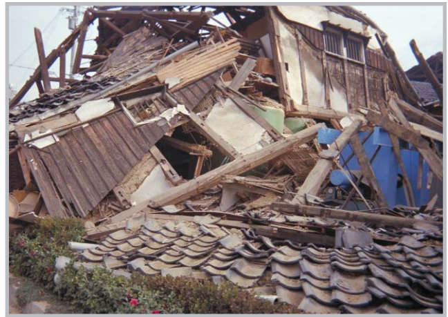
Most fatalities in Japanese earthquakes are caused by the collapse of traditional post-and-beam wooden houses with heavy tiled roofs, as was seen in the 1995 Kobe Earthquake
