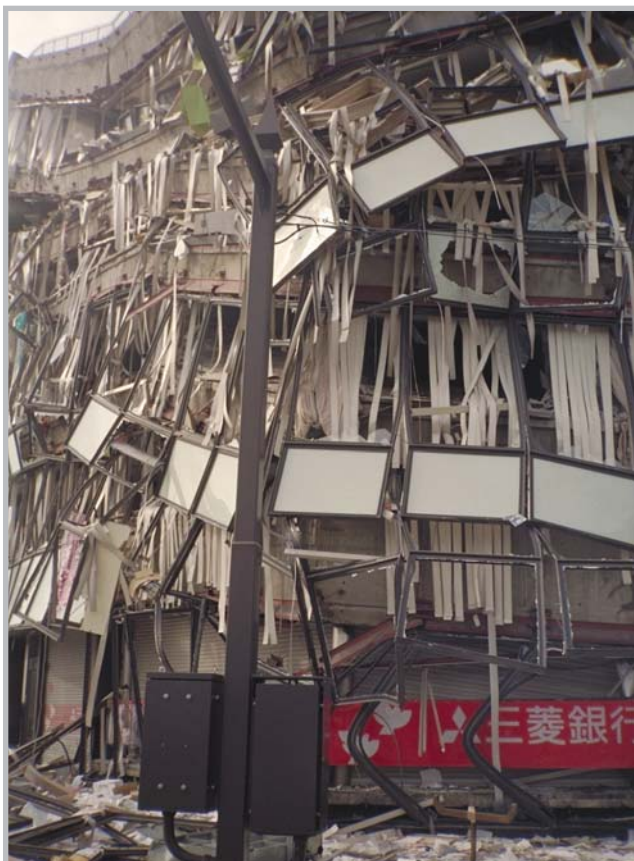
The collapse of multi-story buildings in the 1995 Kobe Earthquake would have killed more people had it occurred during the working hours
