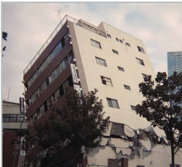
Improvements in building codes failed to prevent the collapse of modern reinforced concrete buildings in the 1995 Kobe Earthquake
