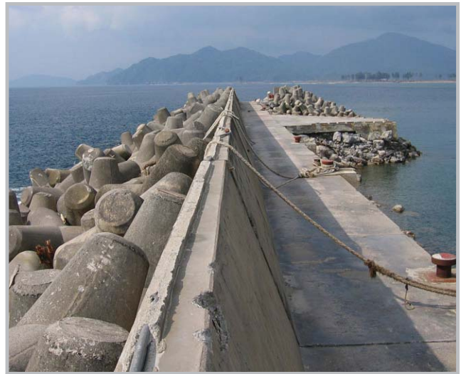
Tsunami walls can provide extra protection against moderate waves, weakening the impact on the urban areas, but are unlikely to withhold larger tsunamis (Source: USGS)
