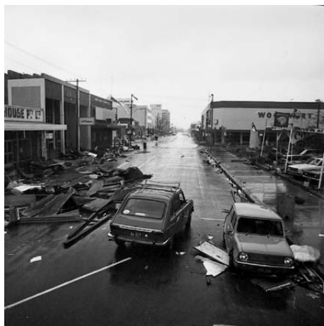
Figure 4: Damage to Smith St., Darwin (NAA)
