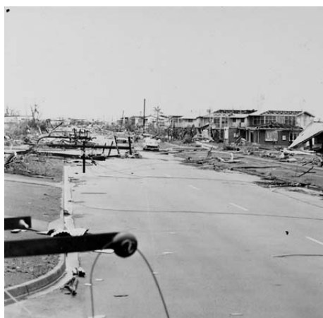
Figure 3: Modern residential neighborhood damage Ross St., Darwin (NAA)
