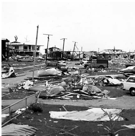
Figure 2: Damage from Cyclone Tracy in the residential neighborhood of Amsterdam Circuit (National Archives of Australia (NAA))
