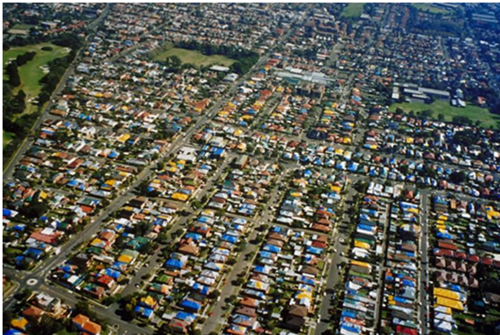
Figure 1: Blue covers on roofs damaged by hail during the 1999 Sydney Hailstorm (Source: Emergency Management Australia)
