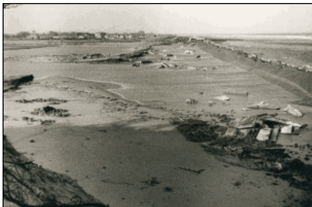
Figure 5. Seawater washed over and broke through walls and earth dikes (Courtesy Professor Wolf)
