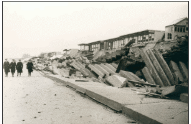
Figure 4. Hard engineered walls and concrete defences were severely damaged by the pounding waves (Courtesy Professor Wolf)
