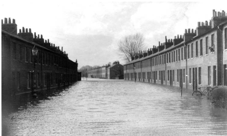
Figure 1: Flooding of Albert Street in Windsor, one of many towns impacted by the 1947 river floods
