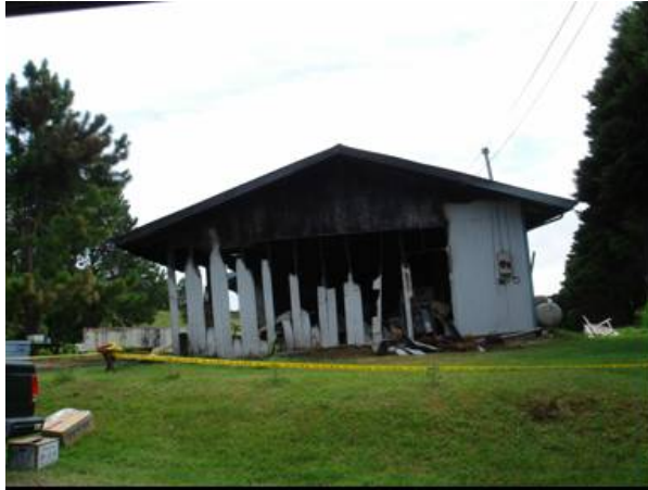
Figure 10: House destroyed by fire following earthquake in Waimea
