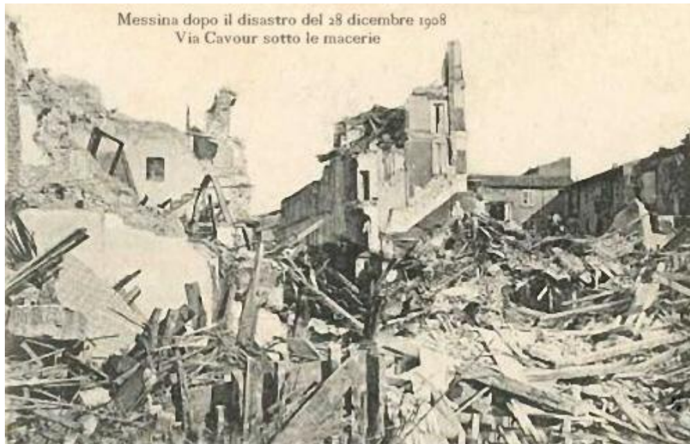
Figure 4: Rubble along the main street of Via Cavour in Messina, Sicily as a result of the 1908 Messina Earthquake (Source: http://www.grifasi-sicilia.com/messina_terremoto_1908_gbr.html )
